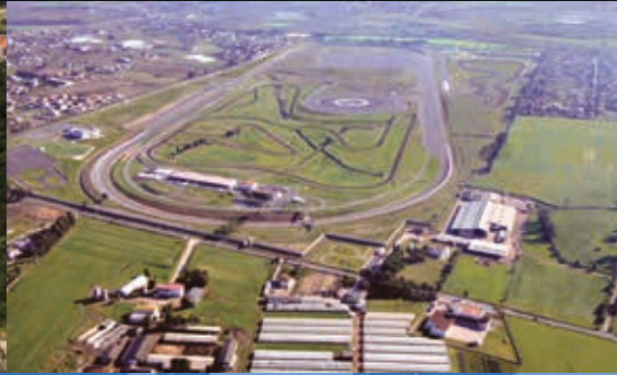
The Bridgestone/Firestone Research & Development Centre ROME.
